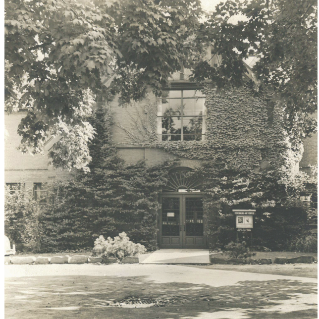
Exterior photograph of Fitchburg Art Museum's original entrance on Merriam Parkway. Photograph from the Fitchburg Art Museum archive
